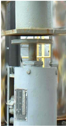
Figure 2 Supports with Questionable Load Capacity
